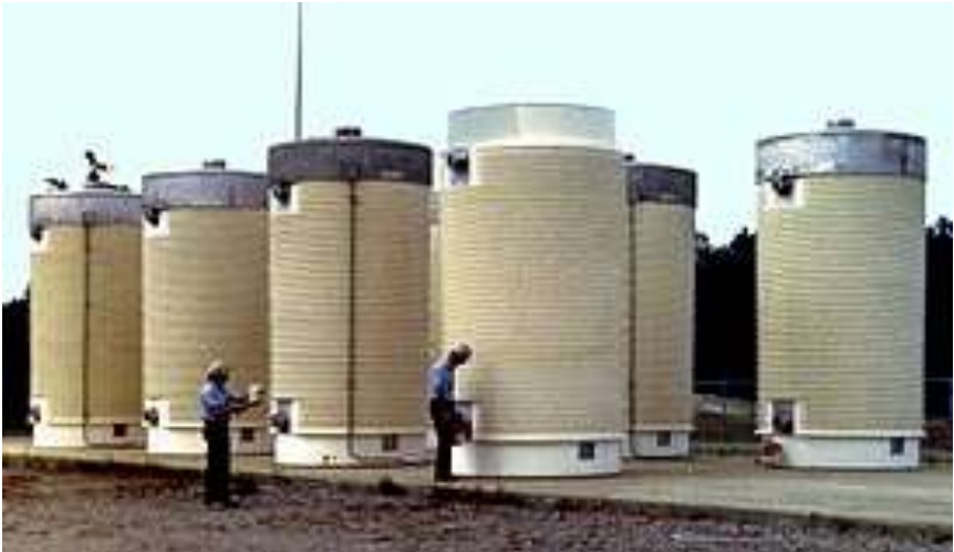
Spent fuel casks. No worker radiation protection is needed.
