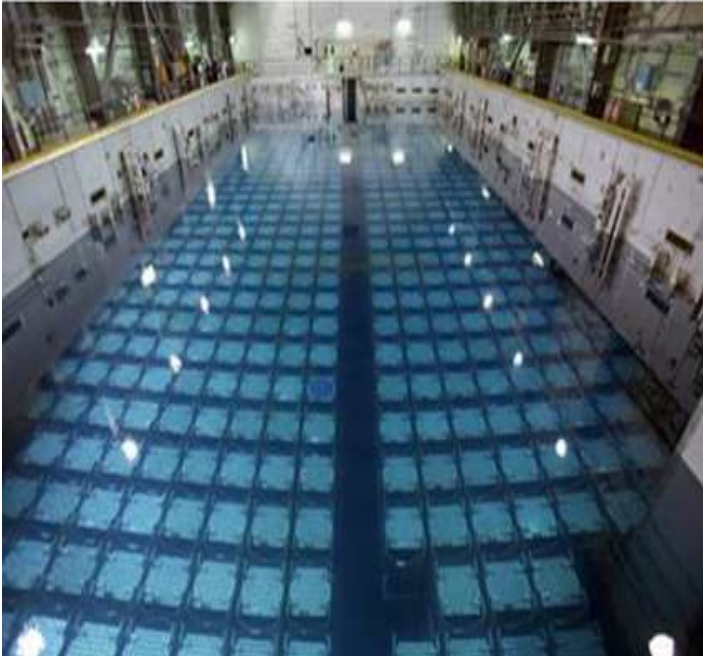
Spent fuel bundles stored in a nuclear plant. Just 3" of water reduces the radiation by 50%.
